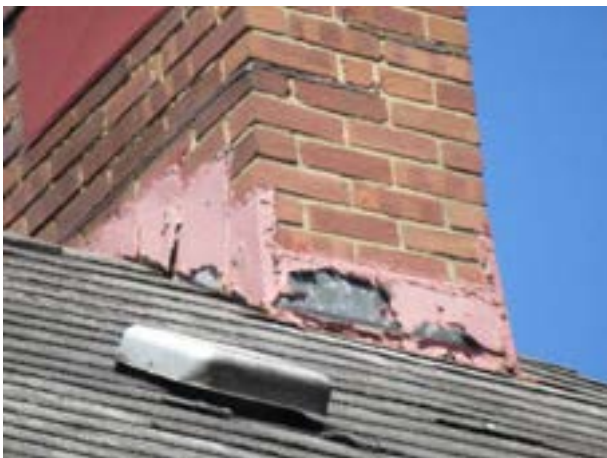
Flashing deterioration
