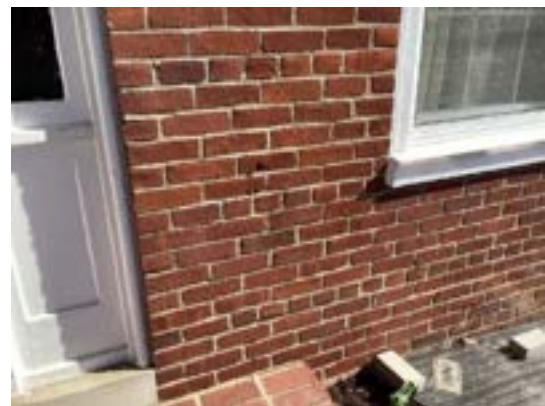
Masonry spall
