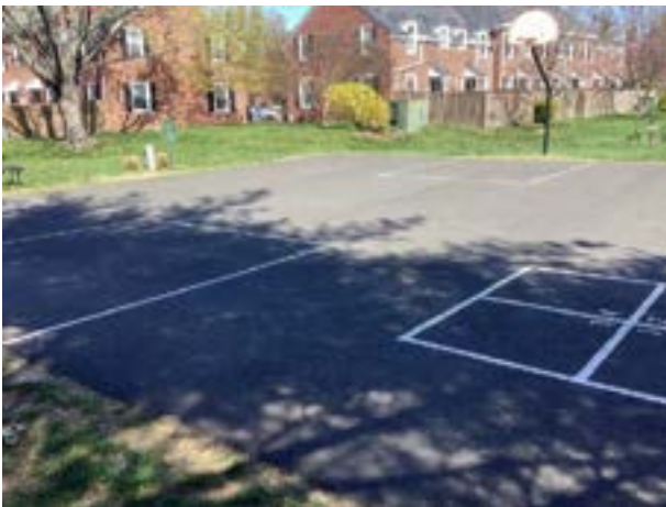
Basketball court overview
