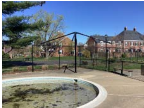
Shade structure overview
