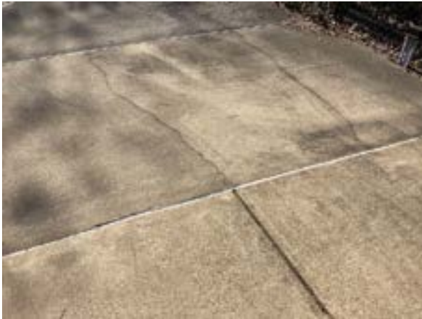
Concrete cracks
