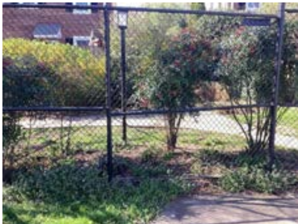
Chain link pool fence
