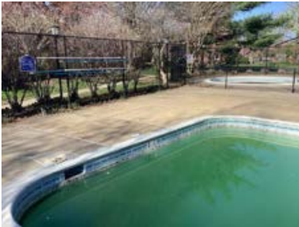
Concrete pool deck overview
