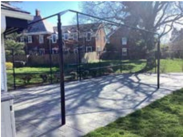
Shade structure overview
