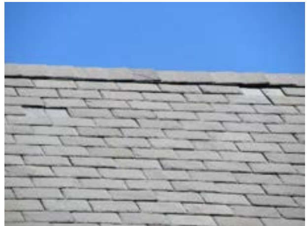
Missing shingles
