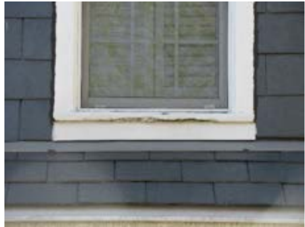
Trim deterioration
