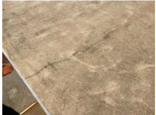
Concrete cracks
