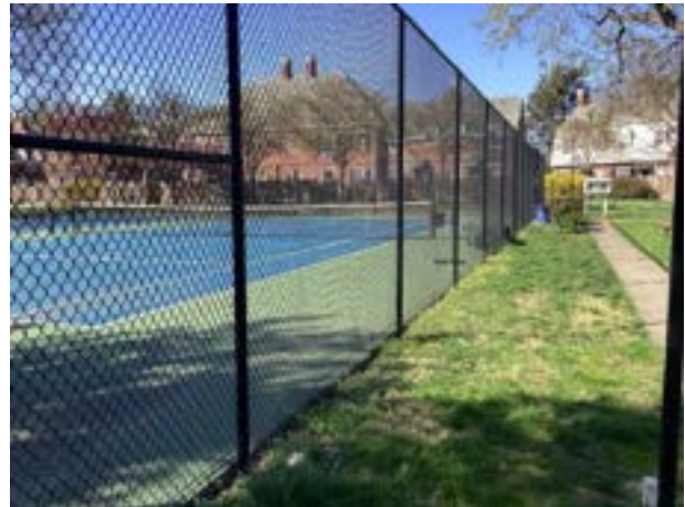
Chain link fence
