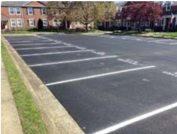
Asphalt pavement parking lot overview
