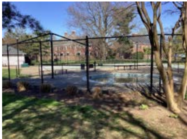
Chain link pool fence
