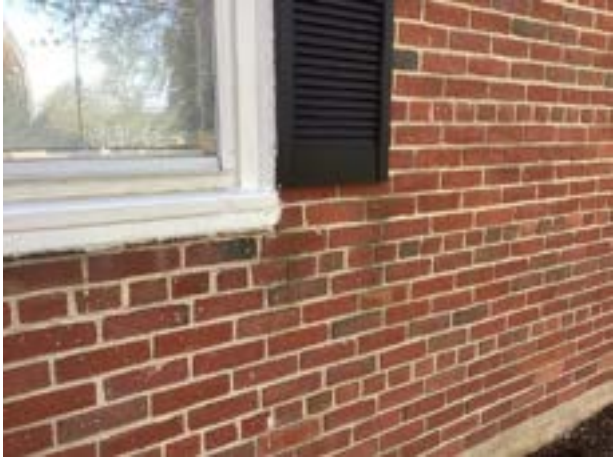
Trim deterioration
