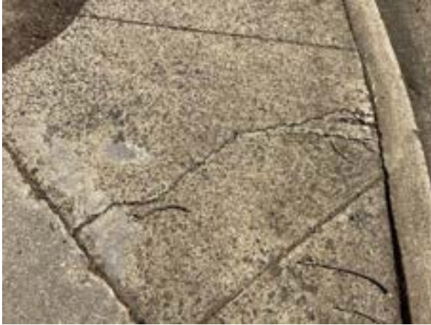
Sidewalk cracks
