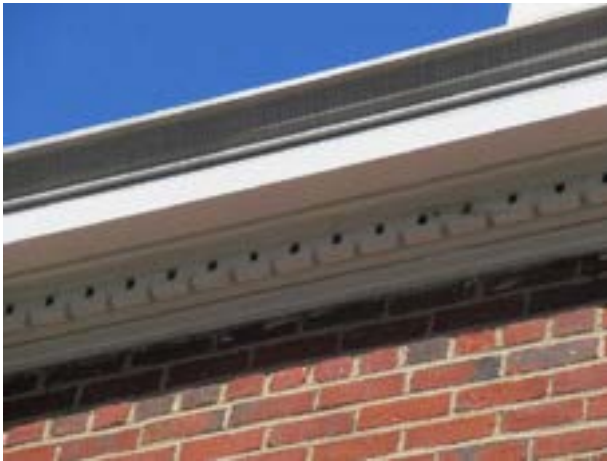
Soffit and fascia overview
