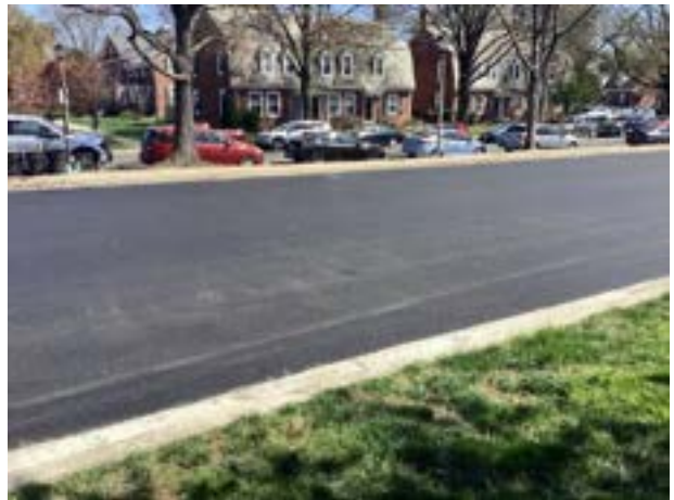
Asphalt pavement parking lot overview
