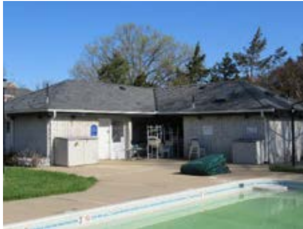
Pool house overview
