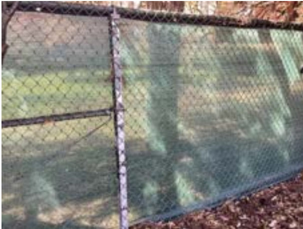
Chain link fence
