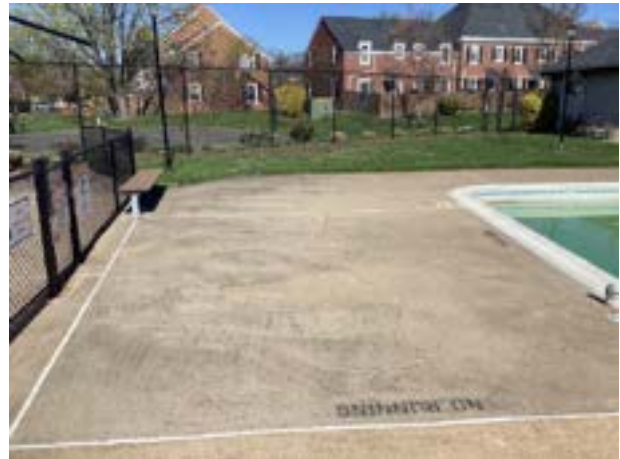
Concrete pool deck overview
