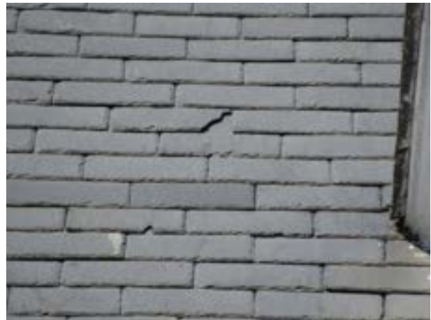
Damaged shingles
