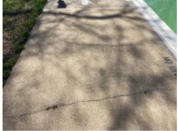
Concrete cracks
