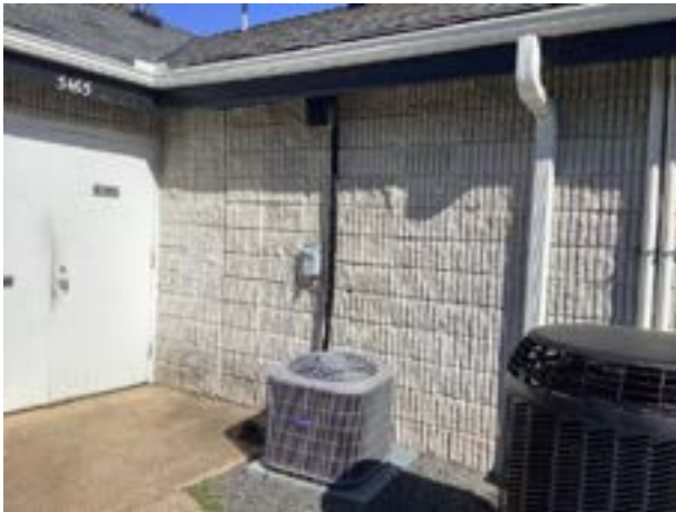
Concrete walls overview
