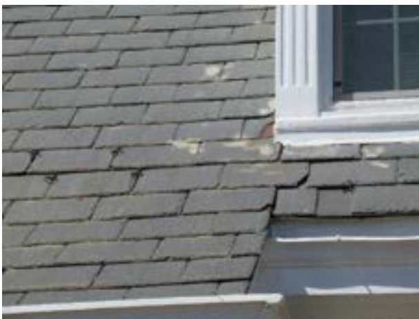
Shingle deterioration
