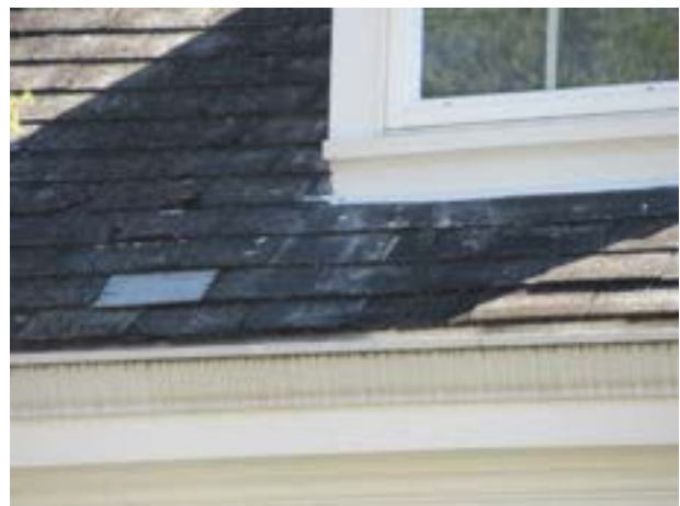
Shingle deterioration
