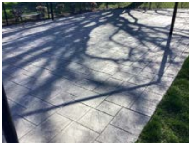
Stamped concrete overview
