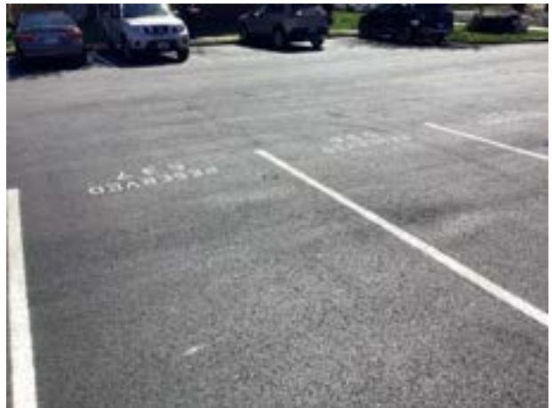
Asphalt pavement parking lot overview
