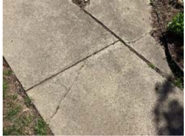
Sidewalk cracks
