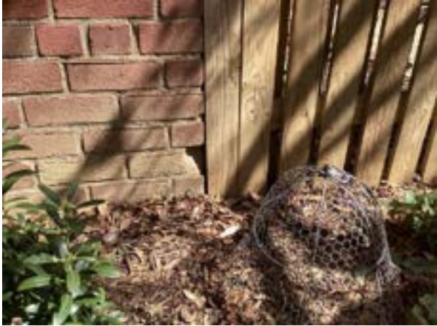
Masonry spall
