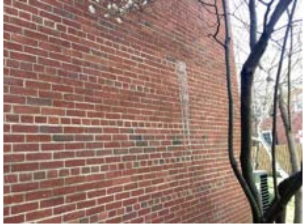
Efflorescence
