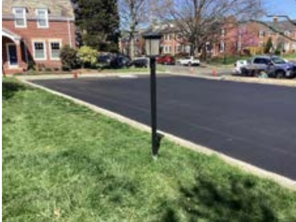
Light pole and fixture
