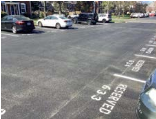
Asphalt pavement parking lot overview
