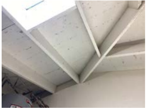
Rest room paint finishes
