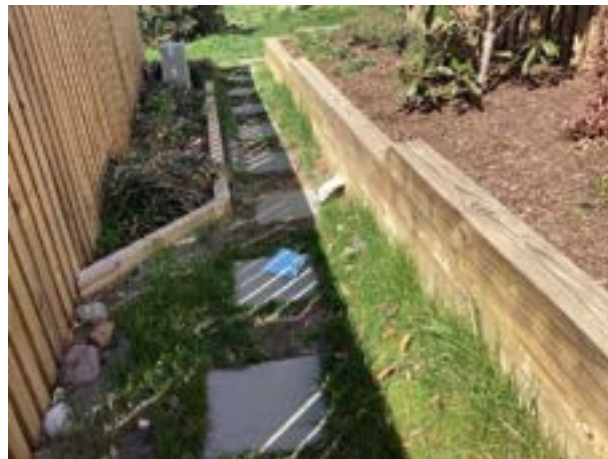
Timber retaining wall
