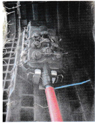
FBOT MOUNTED IN HAND HOLE (FOR ILLUSTRATION PURPOSES ONLY)
