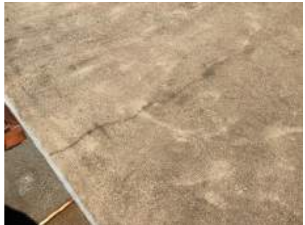
Concrete cracks
