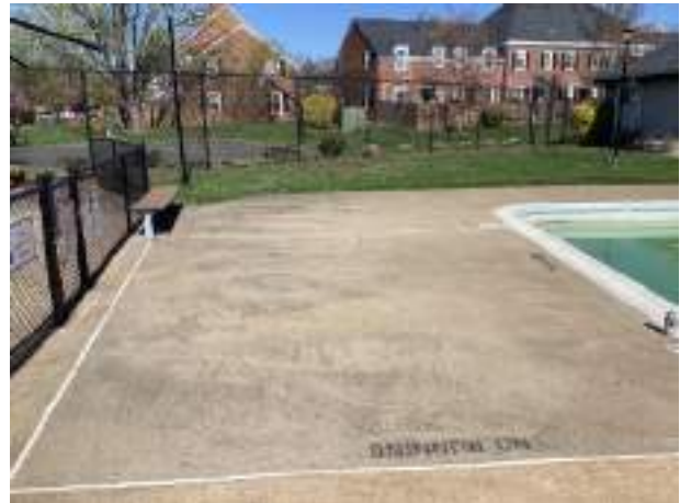
Concrete pool deck overview
