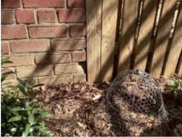
Masonry spall
