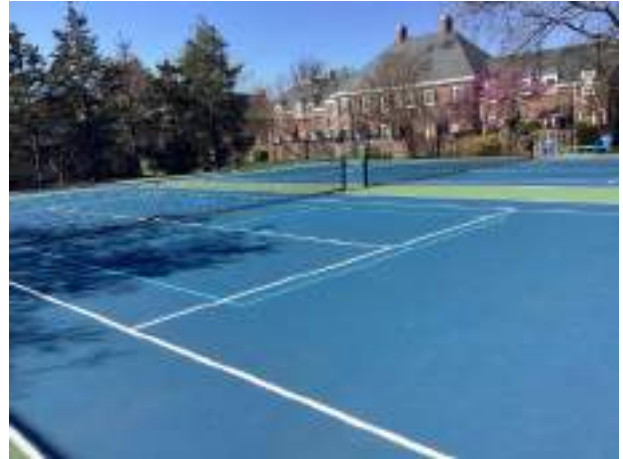
Tennis court overview
