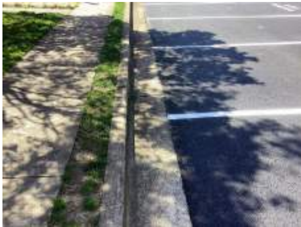
Concrete curb and gutter
