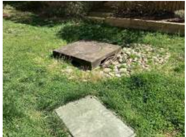
Landscape catch basin
