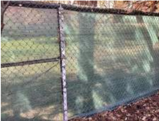
Chain link fence
