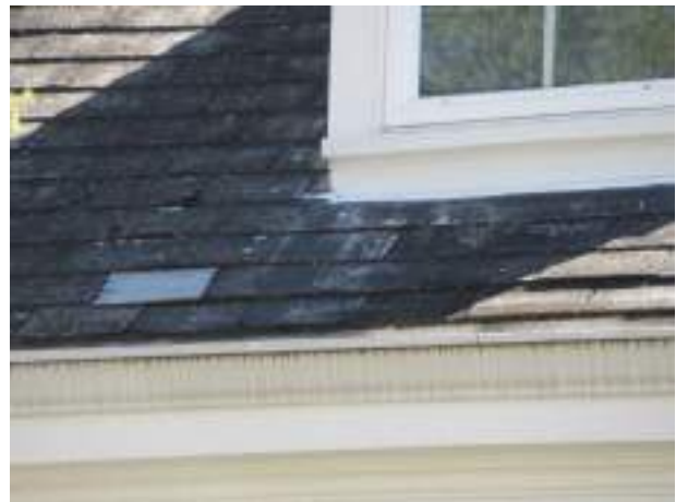
Shingle deterioration
