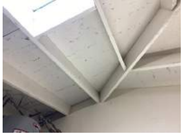
Rest room paint finishes
