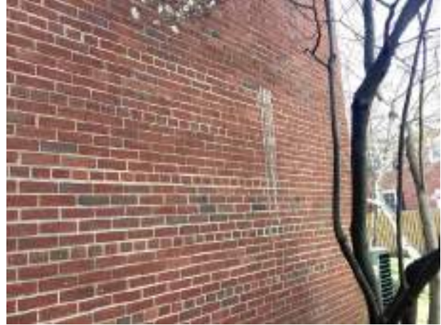
Efflorescence
