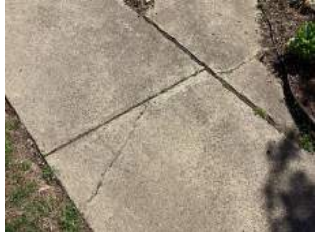
Sidewalk cracks
