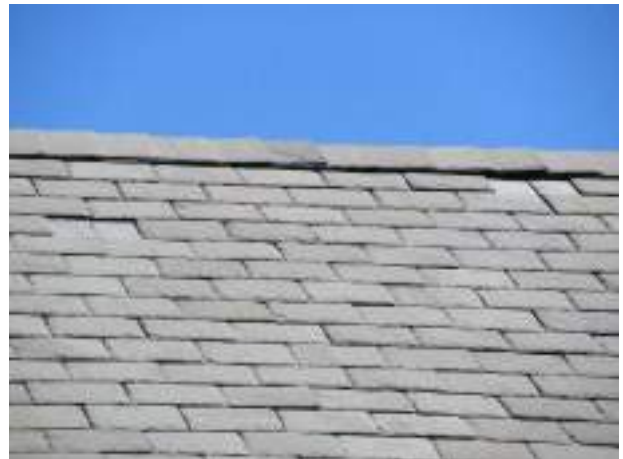
Missing shingles
