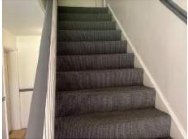
Carpet floor coverings
