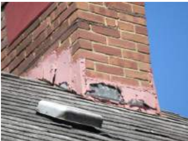
Flashing deterioration
