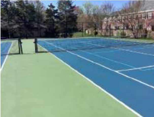
Tennis court overview
