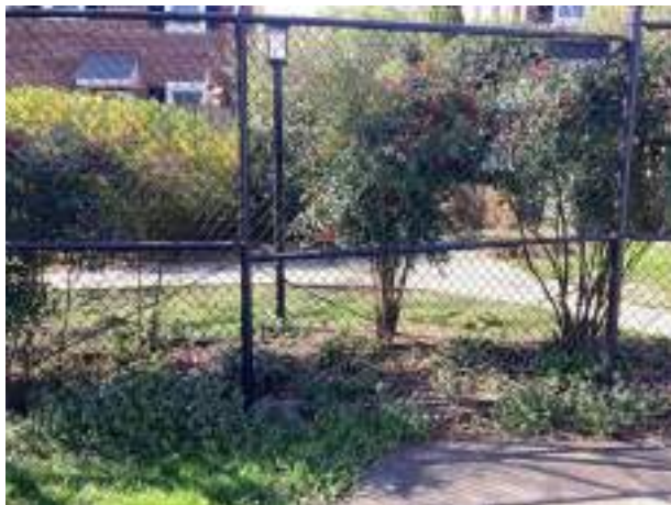
Chain link pool fence
