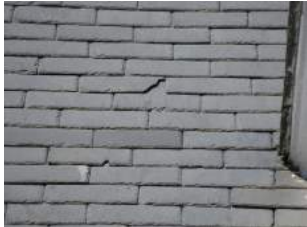
Damaged shingles
