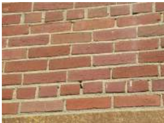
Mortar deterioration
