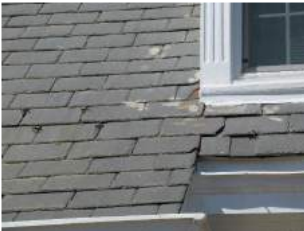
Shingle deterioration
