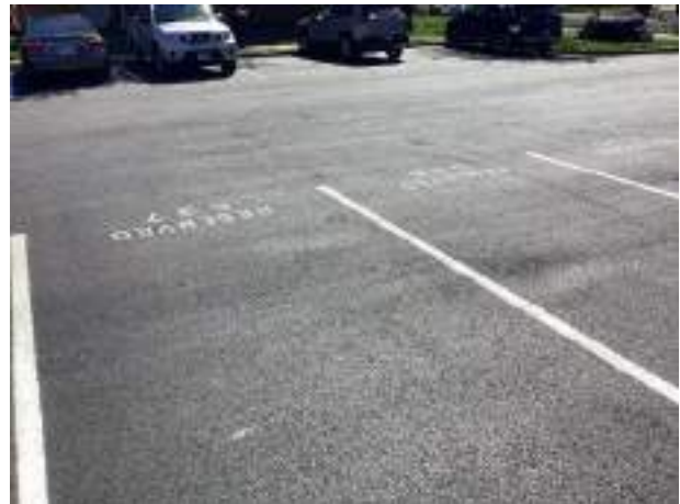
Asphalt pavement parking lot overview
