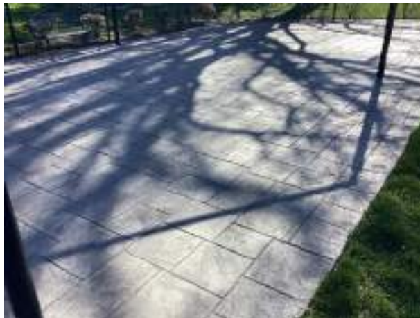
Stamped concrete overview
