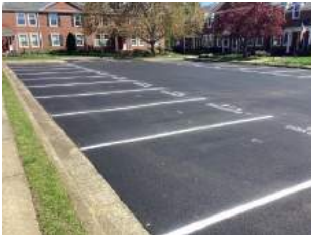
Asphalt pavement parking lot overview
