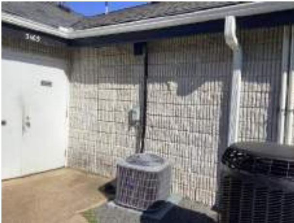
Concrete walls overview
