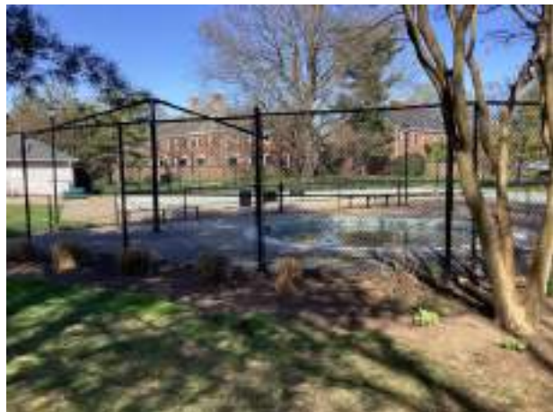
Chain link pool fence
