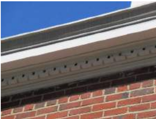
Soffit and fascia overview
