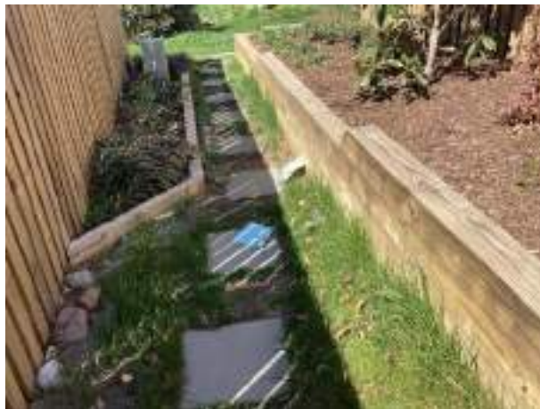
Timber retaining wall
