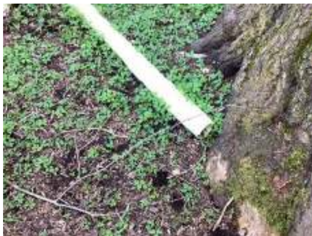
Dented downspout
