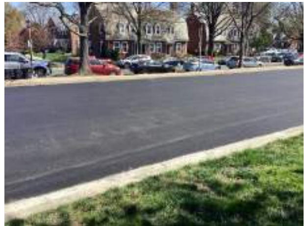
Asphalt pavement parking lot overview
