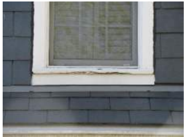
Trim deterioration
