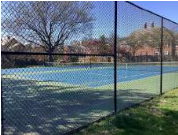
Chain link fence
