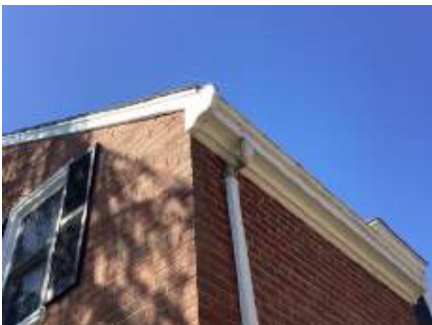
Aluminum gutters and downspouts
