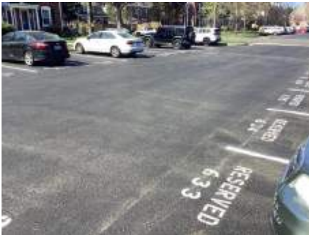
Asphalt pavement parking lot overview
