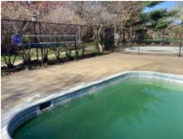
Concrete pool deck overview
