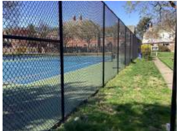
Chain link fence
