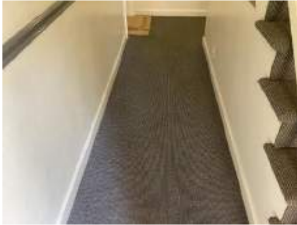
Carpet floor coverings
