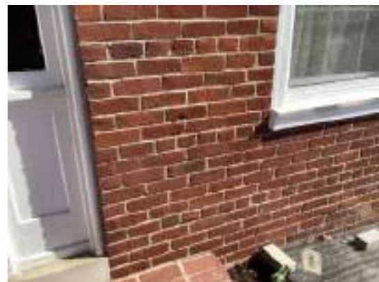
Masonry spall
