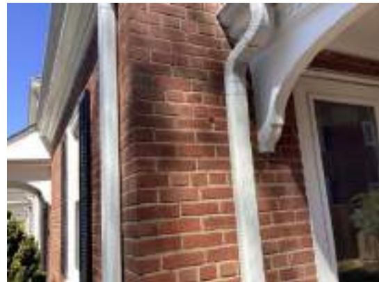
Mortar deterioration
