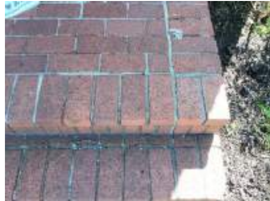
Masonry cracks
