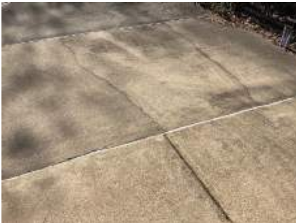
Concrete cracks
